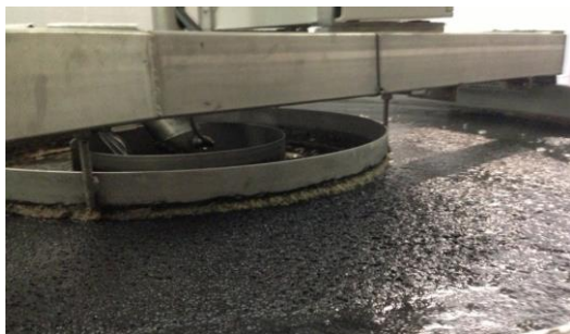
Abbildung 2: Detail Flotationsanlage (A. Langbein).
